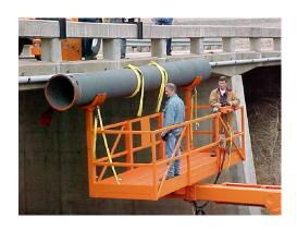
15. Move platform assembly into desired position under bridge and telescope pipe cradle to position pipe.
