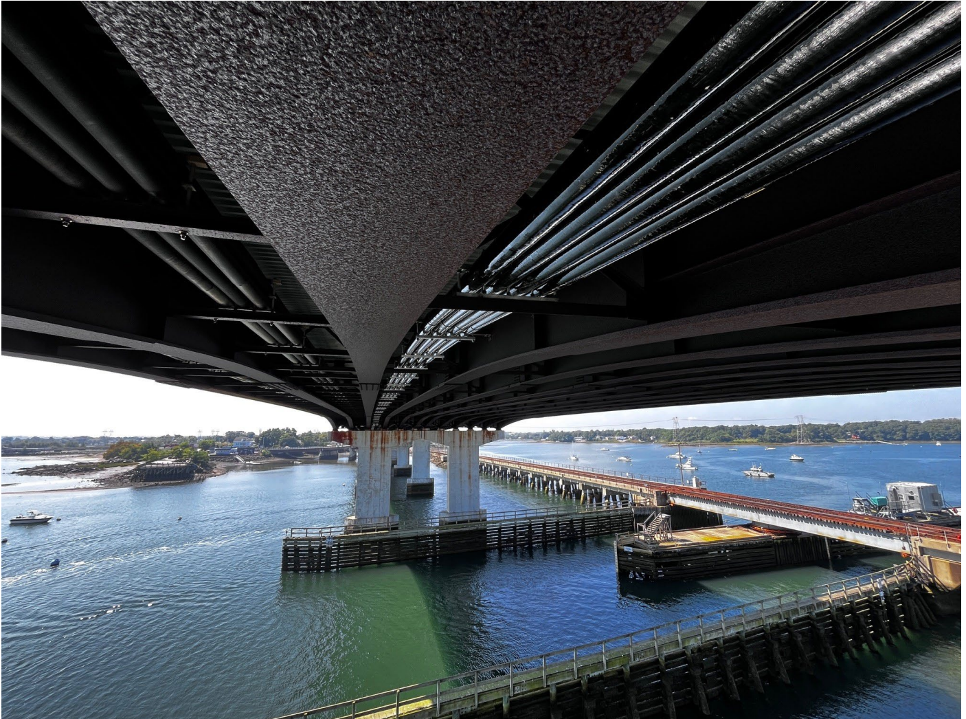
Winona Osborn Essex Bridge - Salem / Beverly, MA
