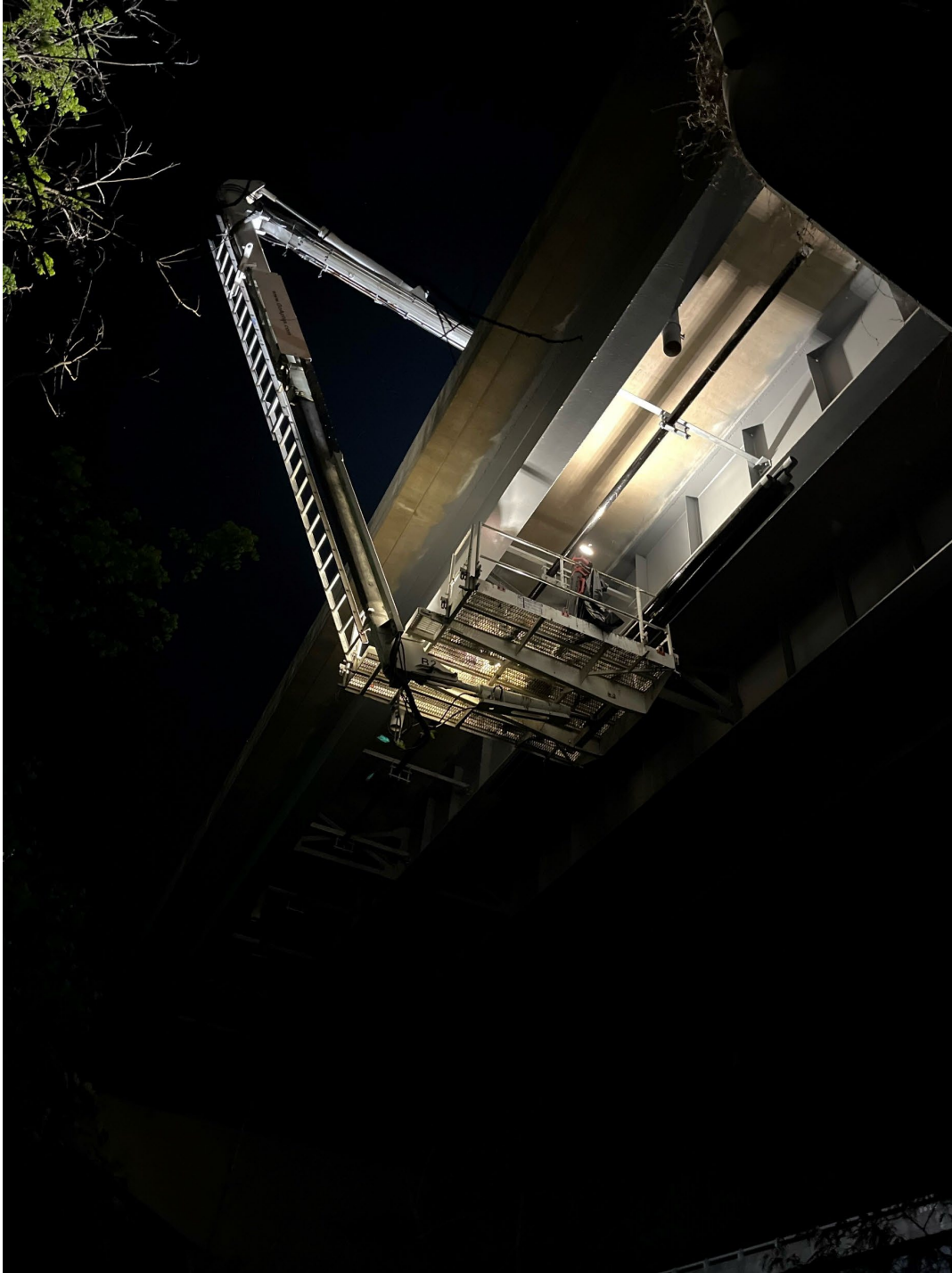
Winona Osborn VA, I-66 Bridge over the Shenandoah River
